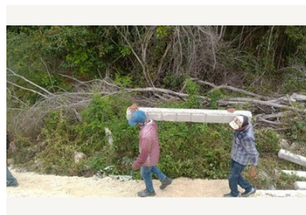
Transport to the work front.
