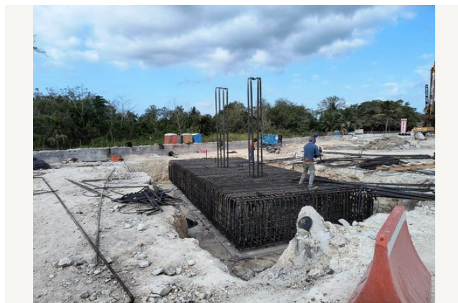
Assembly of foundation reinforcement.
